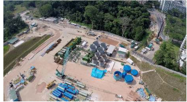
2x1000m 3 /hr Slurry Treatment Plants, Singapore
