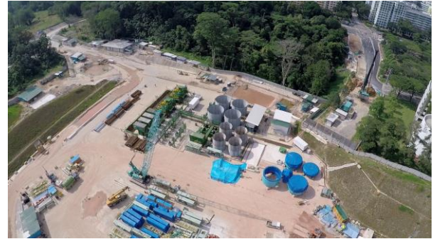
2x1000m 3 /hr Slurry Treatment Plants, Singapore
